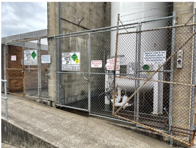
Figure 12- 30kl Gas Tank and Blockwork Enclosure
